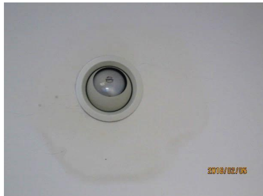
Staining around front recessed lights
