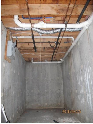
Under utility room
