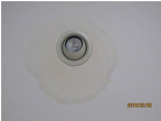
Staining around front recessed lights
