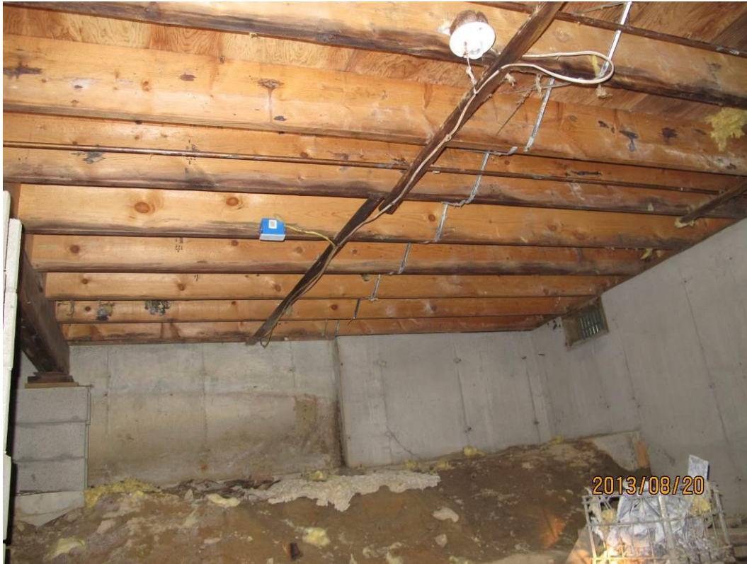
View of left, rear of right crawl space where a third vent is evident that needs to be closed
