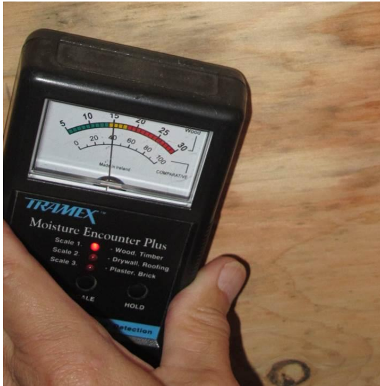
Acceptable MM reading of 15-16% MW in central subflooring
