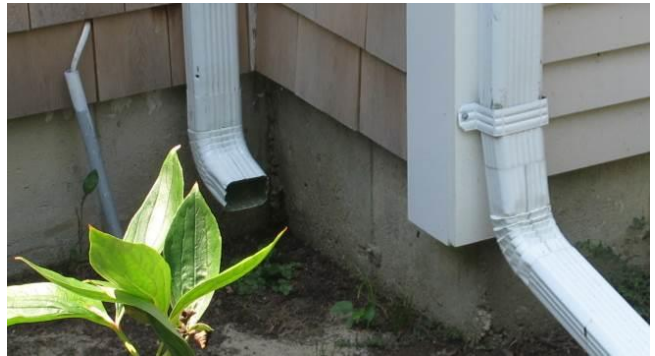
Downspouts discharging too close to the foundation
