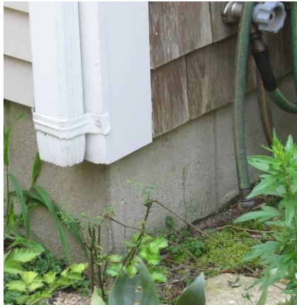
Downspouts discharging too close to the foundation
