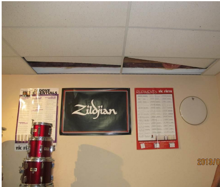
Finished wall in basement against left crawl space [Unknown sized "access" is purportedly behind this wall, perhaps only a third air vent.]
