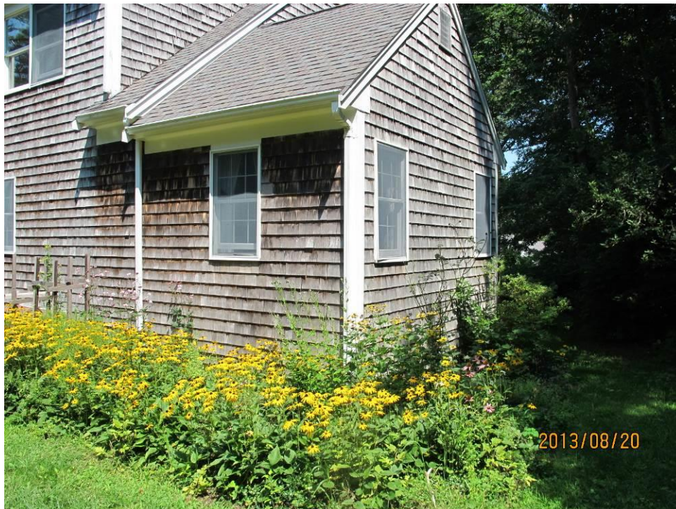
Right master bedroom wing over right crawl space
