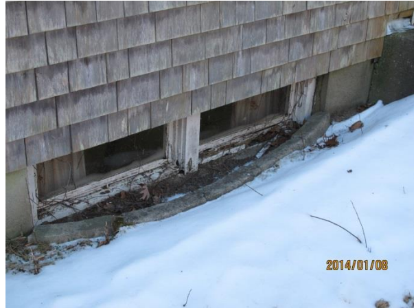
Rotted windows that allow water and outside air to enter the lower level hall
