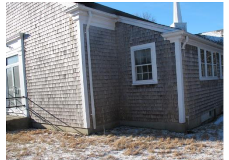
Improperly installed/maintained downspouts that allow water to be discharged at the foundation
