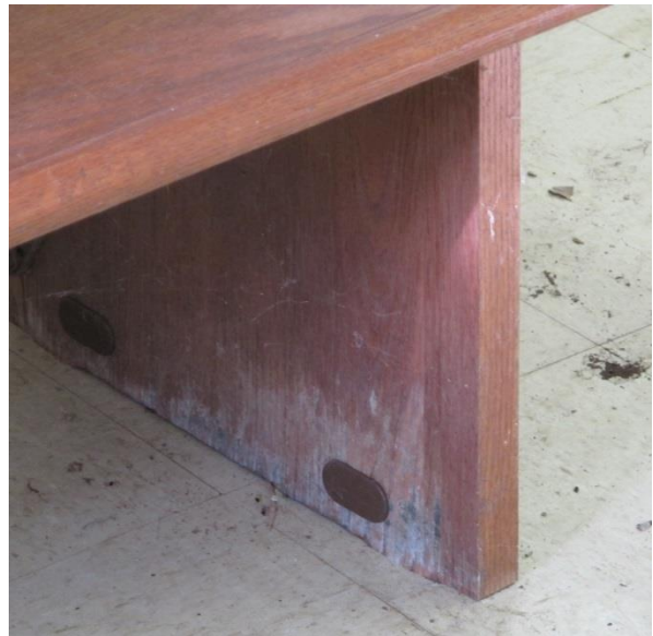
Indication of leaking under south door leading to puddling that affected pew stored nearby (see below)
