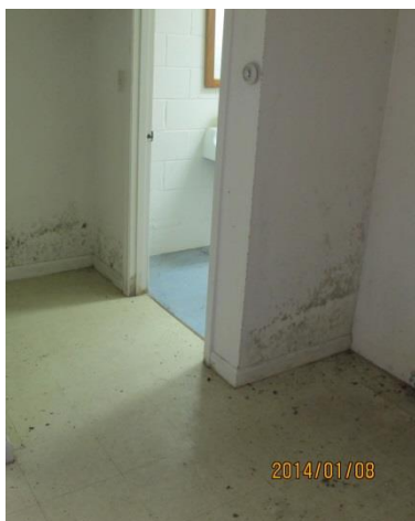
VMG outside men's room near north wall leak
