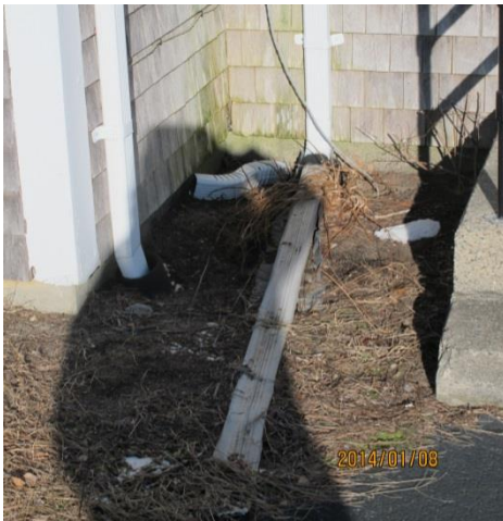
Improperly installed/maintained downspouts that allow water to be discharged at the foundation
