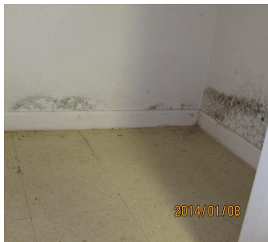
VMG outside men's room near north wall leak
