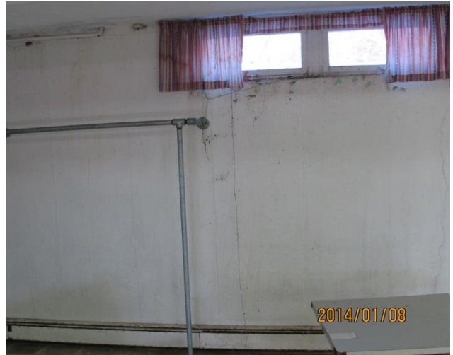
Leaking window on north wall
