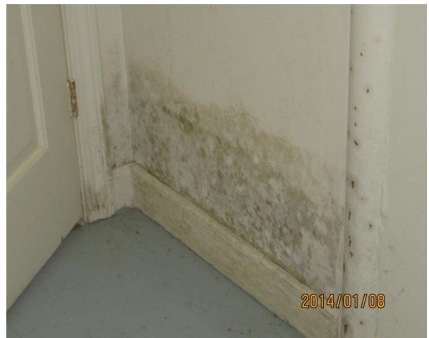
Behind ladies room door (backing on cabinets)
