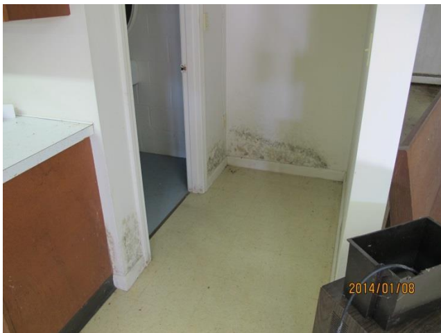
Entry to ladies room
