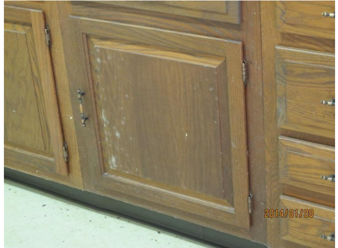
Light CMG on kitchen cabinets (on either side of passage)
