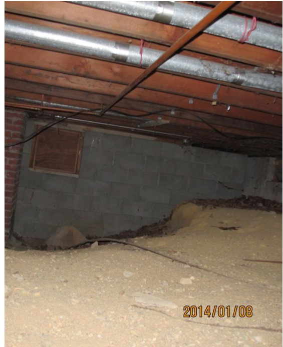
South and north crawlspaces under altar with vents allowing outdoor air to enter
