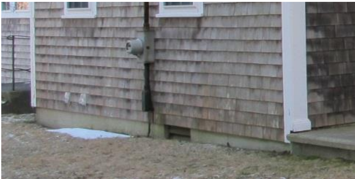
North side vent into the crawlspace under the altar
