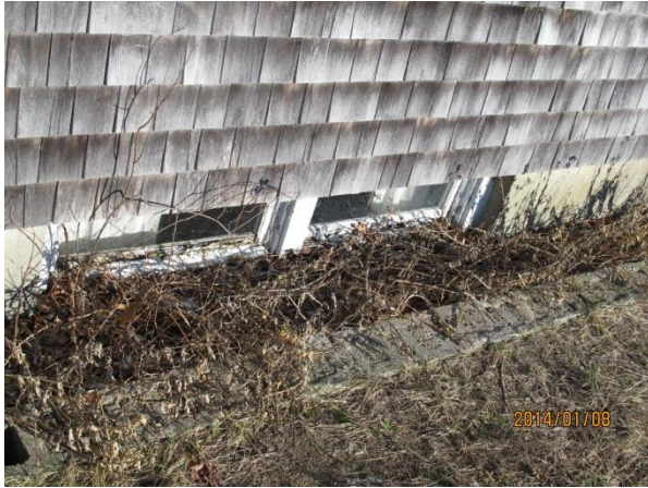
Rotted windows that allow water and outside air to enter the lower level hall
