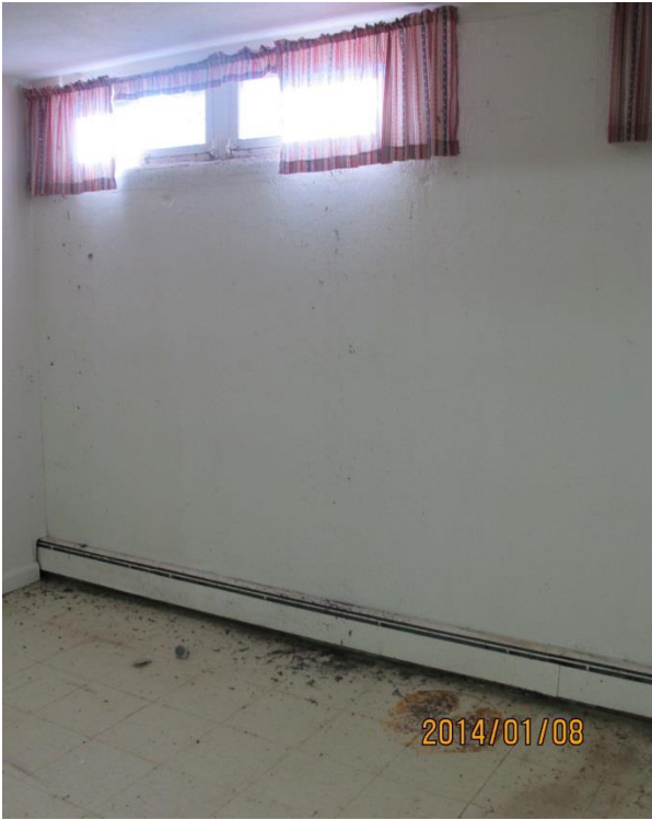
Leaking windows along south wall adding moisture to the lower level
