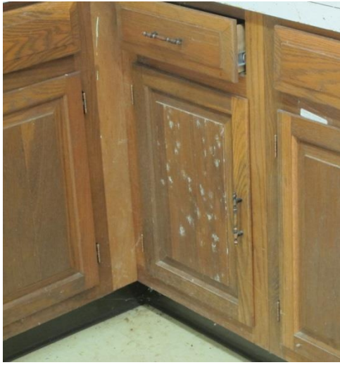
Light CMG on kitchen cabinets (on either side of passage)
