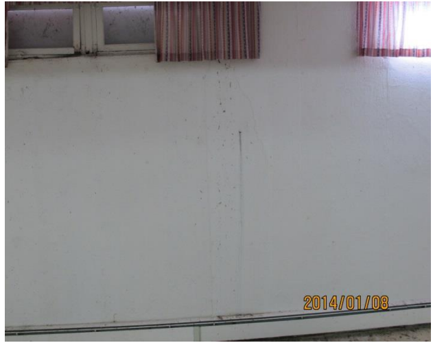
Leaking windows along south wall adding moisture to the lower level
