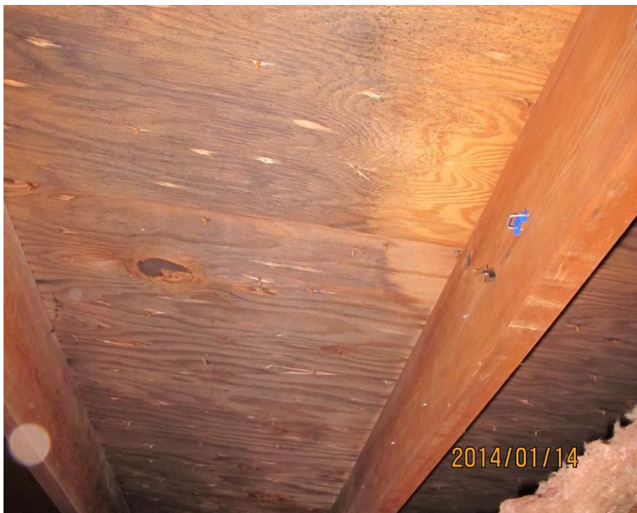
Lighter in-grain mold growth on left side [NOTE cat's eye pattern discussed in Attachment B.]
