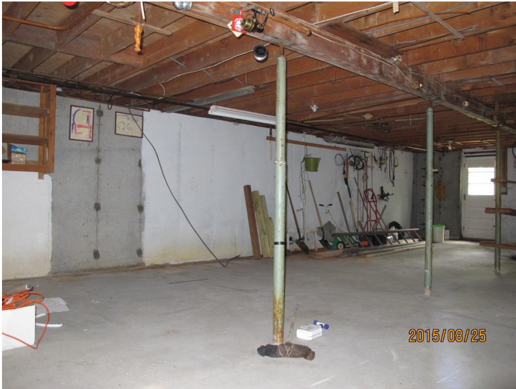
Basement – front wall
