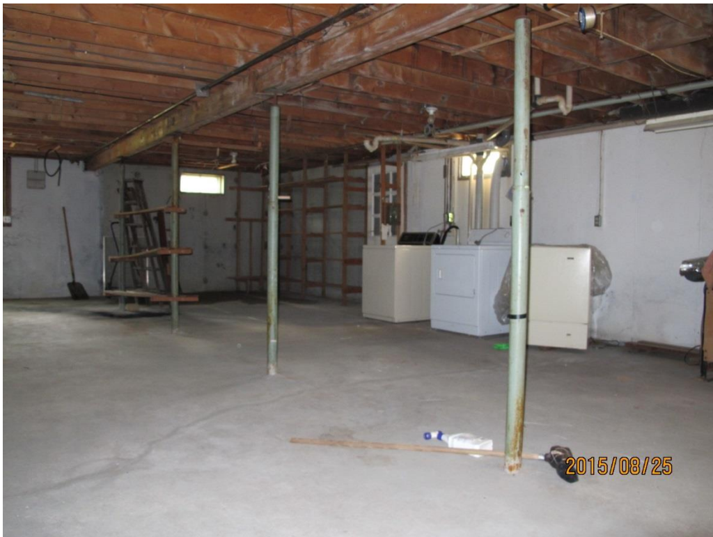
Basement – rear wall
