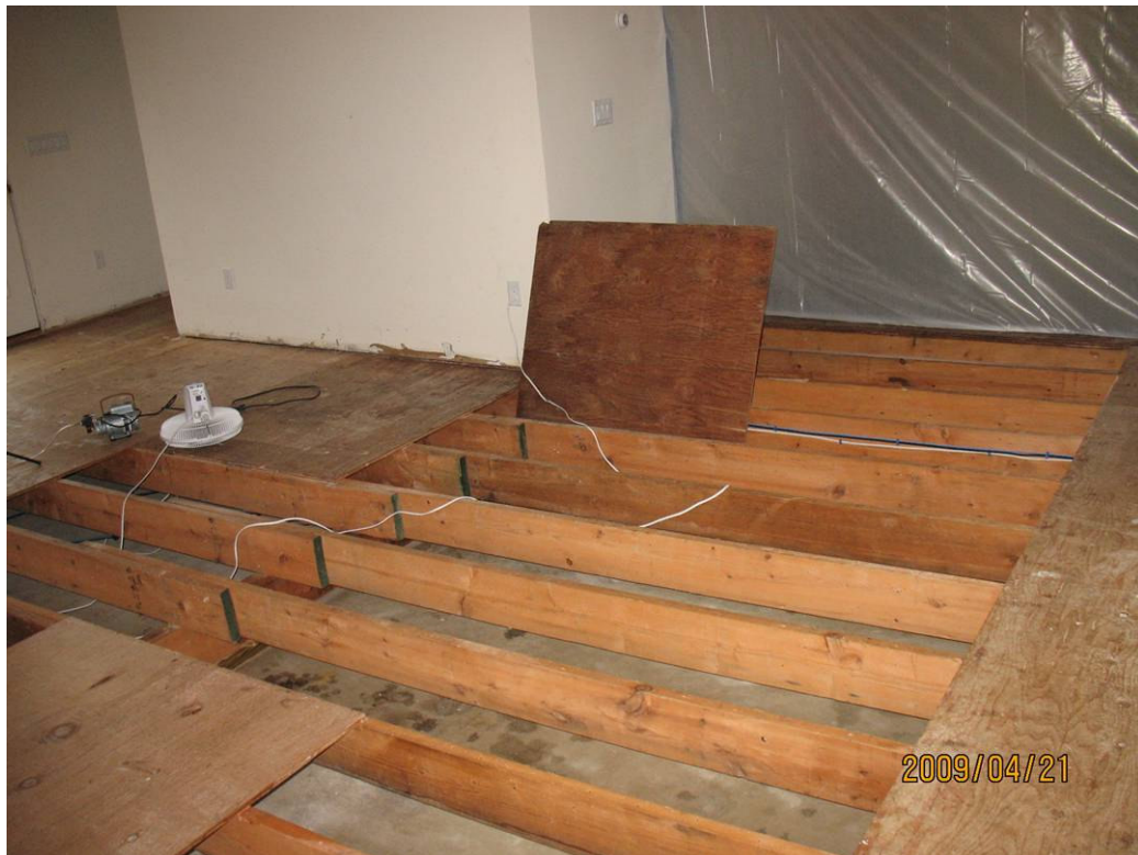
Expanded open floor area in living room.
