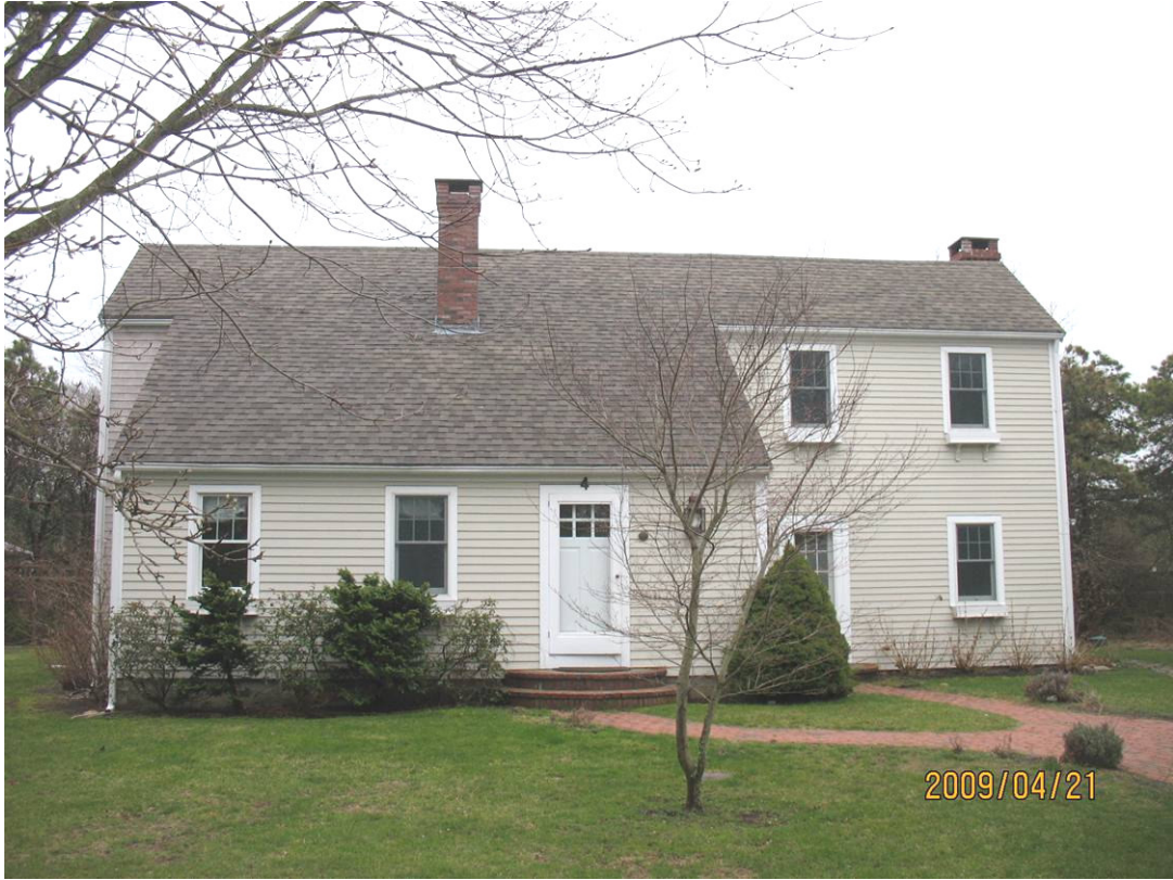
Exterior of house at time of PRV inspection
