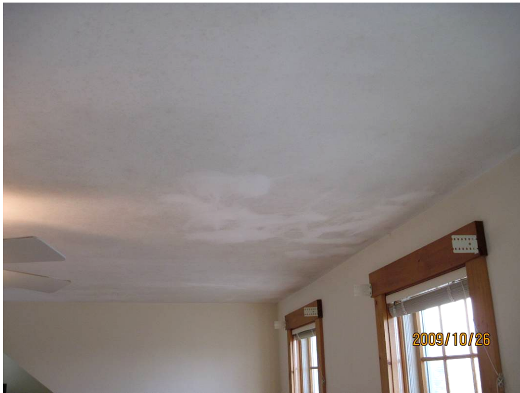
CMG in second floor bedroom where an attempt was made to wipe it off
