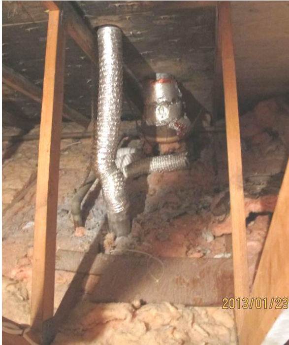
Dryer and shower vents attached properly but without tie-wrap on drying vert.
