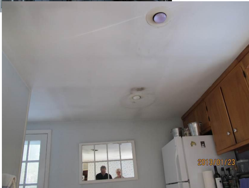
Viewing to east (left) side of kitchen where there is localized VMG near light fixture and linear haze/ghosting
