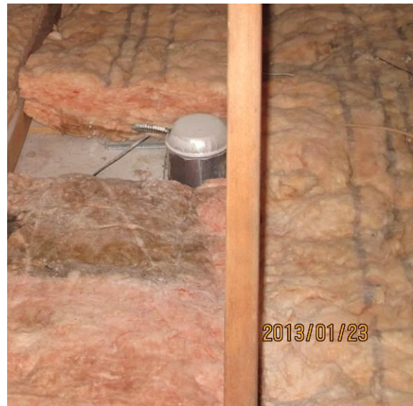
Kitchen ceiling VMG under fixture where insulation had not been replaced
