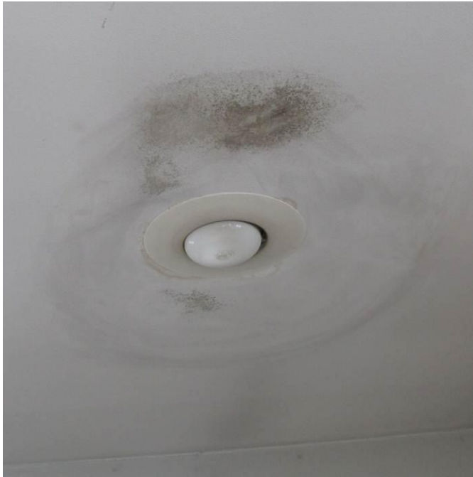
Kitchen ceiling VMG under fixture where insulation had not been replaced [Note are in foreground where insulation had been lifted up over a piece of wood, reducing the insulation of the ceiling and leading to an area of hazing/ghosting
