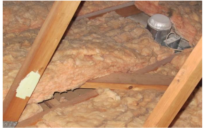
Kitchen ceiling VMG under fixture where insulation had not been replaced [Note are in foreground where insulation had been lifted up over a piece of wood, reducing the insulation of the ceiling and leading to an area of hazing/ghosting
