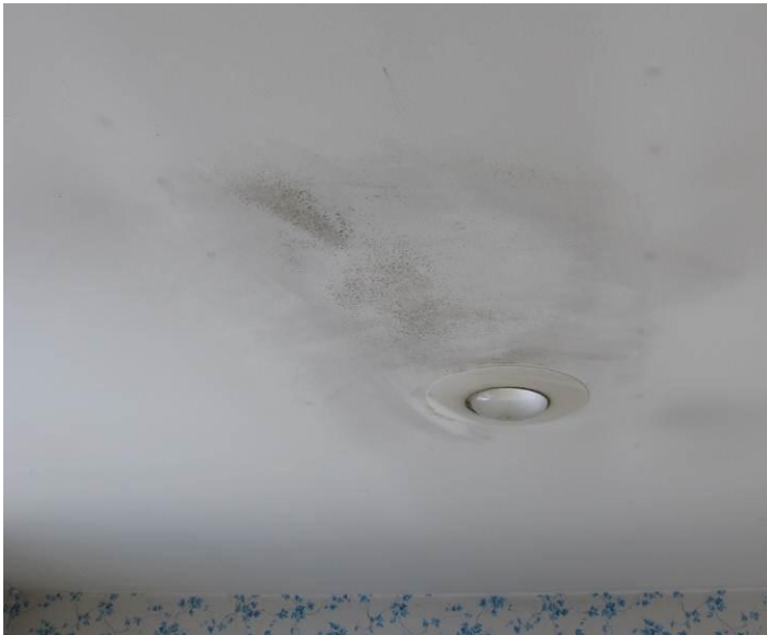
Kitchen ceiling VMG under fixture where insulation had not been replaced
