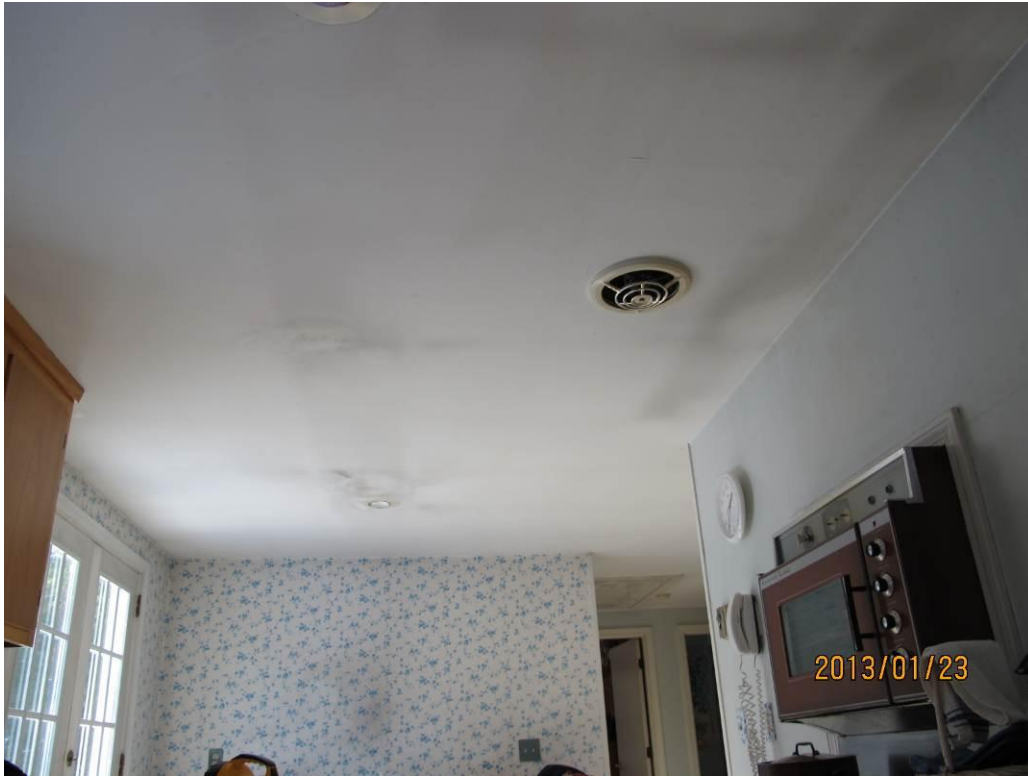
Viewing to west (right) side of kitchen where there is localized VMG near light fixture and linear haze/ghosting
