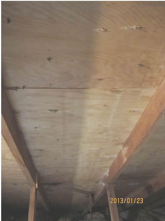
Clear 17-year old sheathing on south (rear) sheathing as opposed to darkened north side sheathing
