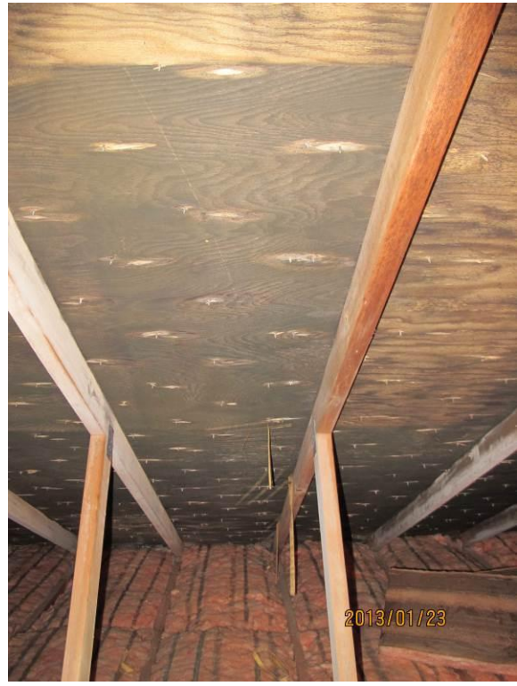
Clear 17-year old sheathing on south (rear) sheathing as opposed to darkened north side sheathing
