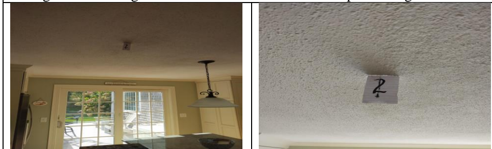
Kitchen Ceiling – distance view to left and close-up to the right
